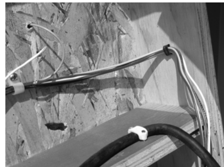
Underside of module showing wires secured for safety purposes
