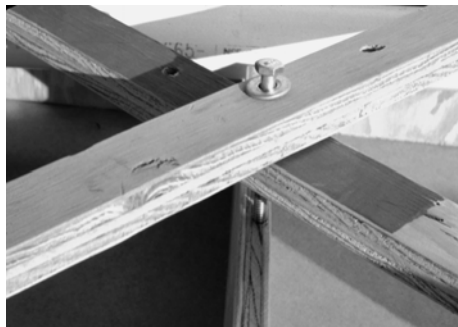
Leg diagonal braces secured for transport
