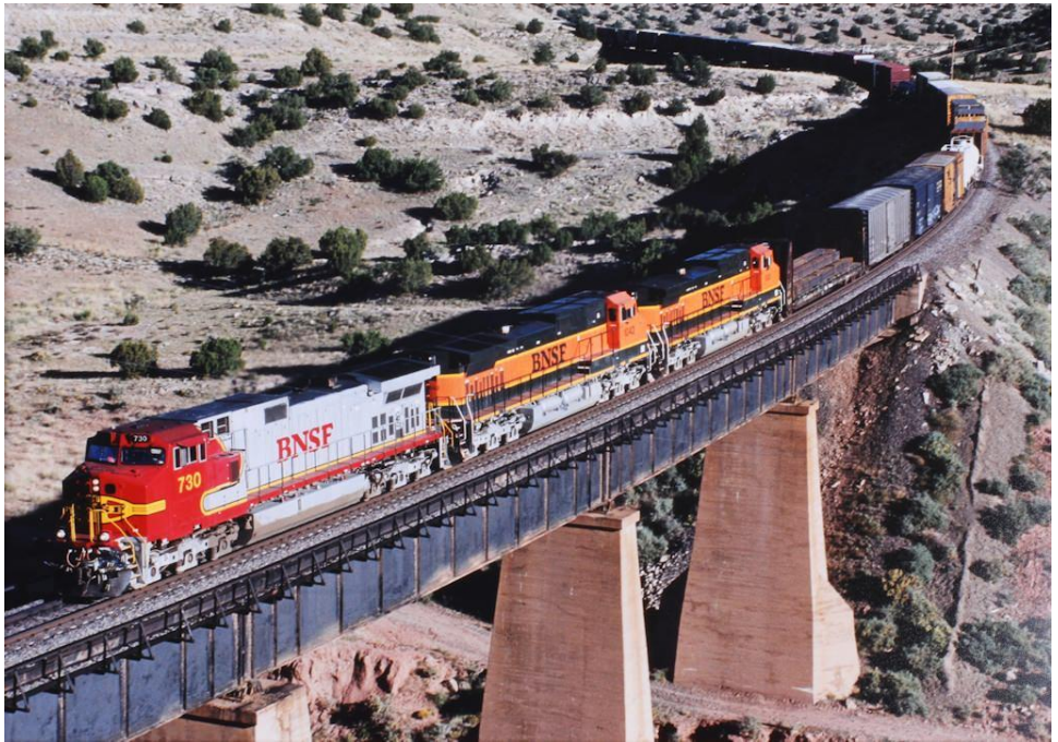
Prototype Photo 2 nd Place: BNSF Over Bridge – Ed Walton
