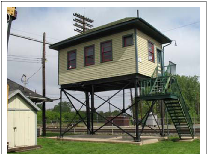
Photo 4. This is the former Erie Railroad AC (Atlantic Crossing) Tower, which has been moved from its original location across the tracks to the Marion Union Station museum site on the south side of the junction. It served the interlocking from 1902 to 1995, and was built on a two story tower instead of the current one-story tower. The tower closed in January 1995 and was moved in November, 1999, and still has the original Taylor Model 2 "pistol-grip" electro-mechanical interlocking machine. AC has been beautifully restored inside and out.
