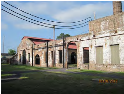
Outside walls of repair complex illustrating the "Savannah gray brick".
