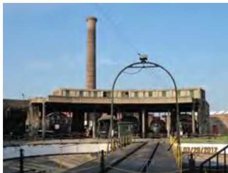
Busy remainder of roundhouse with working 85' turntable.
