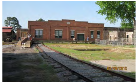
Another repair shop area undergoing restoration (look right).
